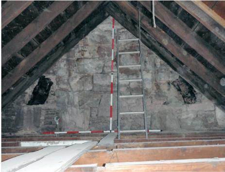
Plate G. Structure 1, loft, chimney flues found in eastern gable.
