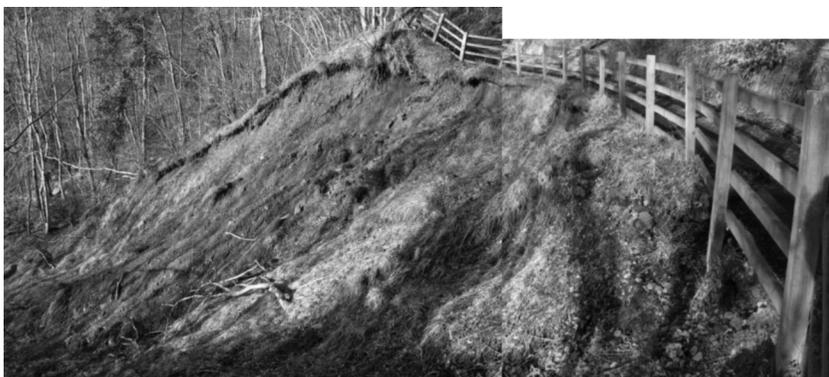
Figure 1. Landslide 1 (numbered approaching from down-valley): This shows new erosion with a debris flow (left), and encroachment on the road pavement (right and below, Figure 2).
