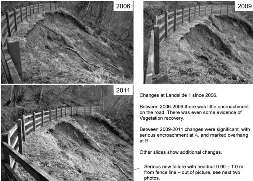
Figure 5. Changes at Landslide 1 since 2006.
