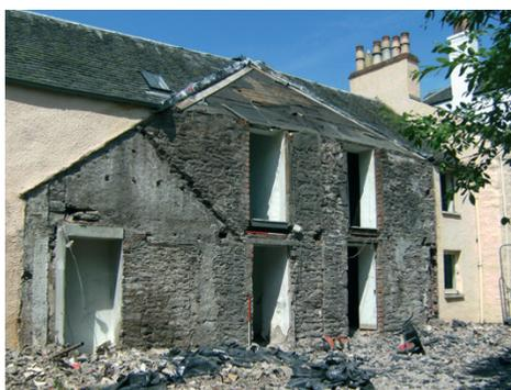
Plate B. Southern external elevation after removal of extension.
