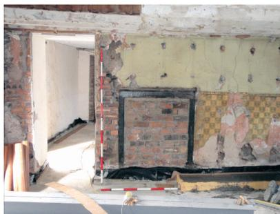
Plate F. Structure 1 ground floor, inserted doorway and blocked fireplace in western elevation.
